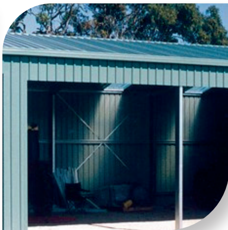
Open Bay Garage
