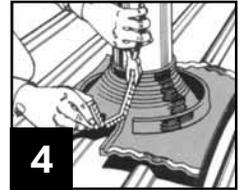
4 Crimp the top three clips with pliers. To assist in completion of crimp, place hand behind the seam for support and continue crimping. Do not overcrimp.
