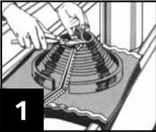
1 Measure outside pipe diameter and trim cone exactly where indicated.
